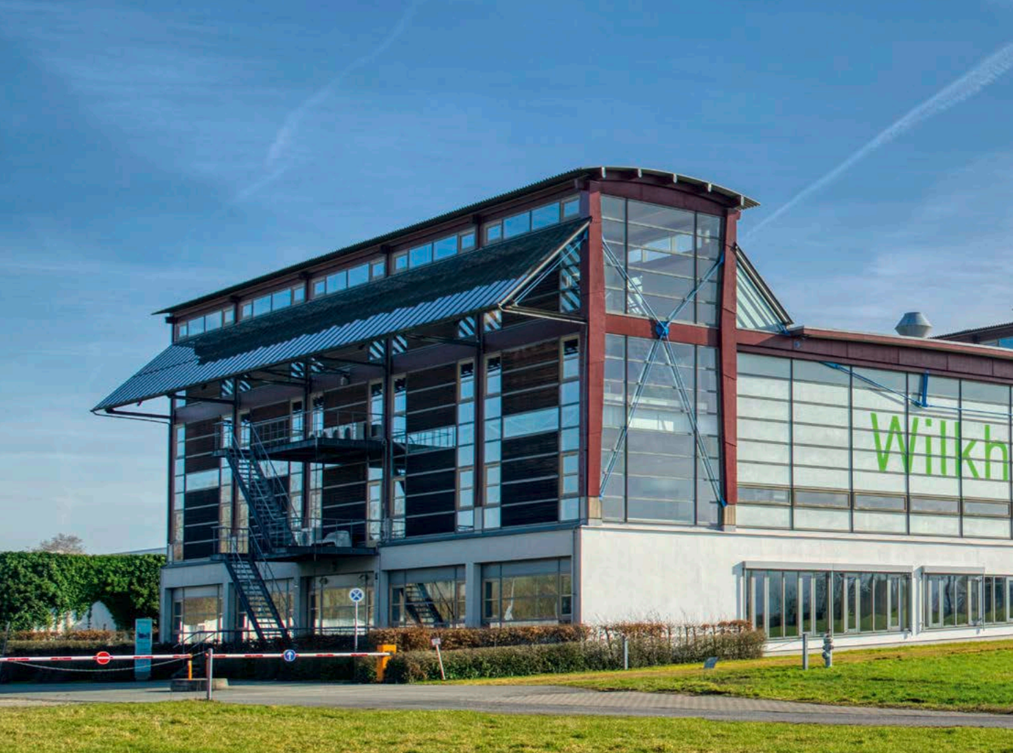
The group of production facilities is visible from afar and stands for the essential qualities of long-lasting product design: authentic materiality, sophisticated construction and a detailed aesthetic.
